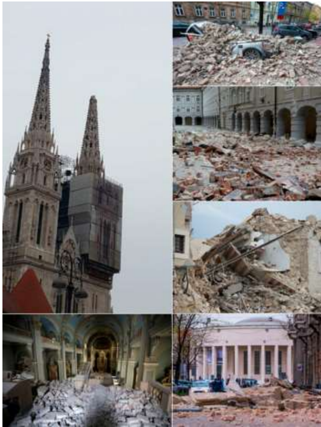
Figure 1. Photos of damage in Zagreb caused by the 22 March 2020 earthquake (from Markušić et al, 2020).
