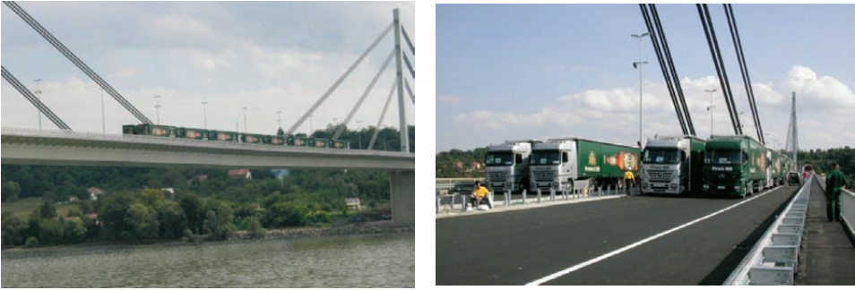
Figure 8. Trial static load.
