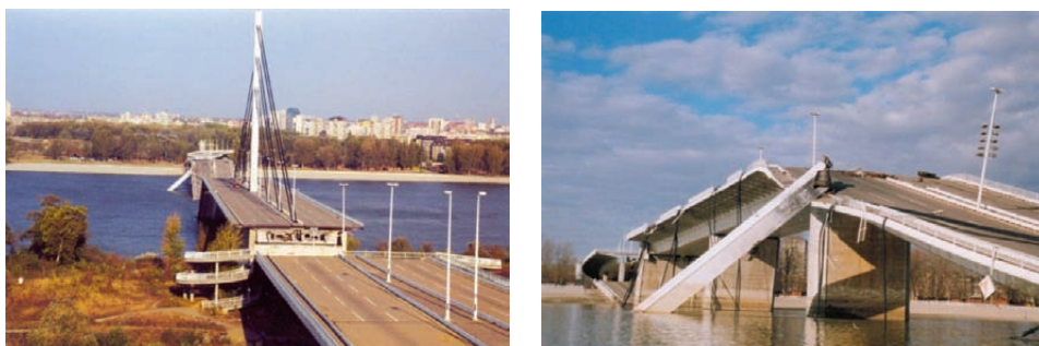
Figure 1. Damaged bridge structure.
